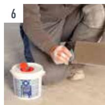
**6** The crack is friction-sealed and closed within 30 minutes. The top cover installation can be continued. Clean tools immediately after use with the cleaning cloths of the UZIN Clean-Box.
