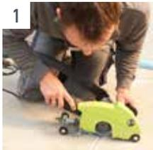
**1** First widen the cracks to allow UZIN KR 516 to be easily poured into them. Treat cracks extending through the entire thickness of the screed by cutting cross-cuts down to 2/3 of the screed depth spaced approx. 25 cm apart; use an angle grinder for this purpose (e.g. Wolff screed groove cutter EF 135).
