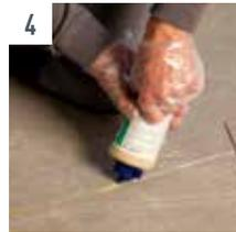
**4** Completely fill the crack with the mix. Level excess resin along the cracks or joints using a trowel with a small width.
