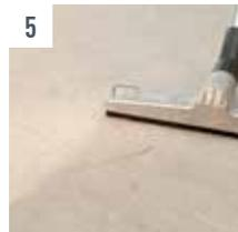
**5** Sand introduced resin with UZIN Silica Sand 0.8 while still damp to achieve a good bond with subsequent materials. Vacuum off loose sand after setting.
