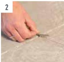
**2** Remove loose edge debris of the screed. Carefully vacuum joints and cracks. Insert the enclosed corrugated links into the cross-cuts.
