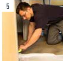
Apply the fibre-reinforced solution adhesive UZIN KE 66 after 1 hour – allowing it to partially dry – using a suitable notched trowel.
