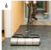
Install the luxury floor covering and roll down once over the whole surface, e.g. using the Wolff pressure roller.
