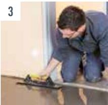
Apply the rapid levelling compound UZIN NC 172 BiTurbo directly onto the surface. The raking method can be used as an alternative to levelling. The screed rake from the UZIN product offering is recommended for this purpose.
