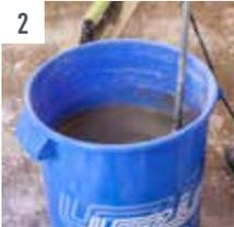
Mix the rapid levelling compound UZIN NC 172 BiTurbo with clear cold water. Use a powerful electric handheld mixer for mixing, e.g. the Wolff agitator Power X 1300.
