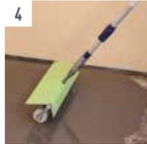
Now use the UZIN spike roller, adjusted to the thickness of the levelling compound, for aeration.
