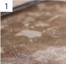
Remove existing floor covering. Sand/brush subfloor to remove flooring remnants and weakly bonded adhesive residues. Thoroughly clean area with a strong industrial vacuum cleaner.
