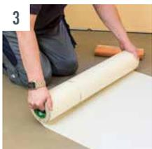
**3** Now perform trial bonding. Rub down Sigan 1 well on the substrate and check whether Sigan 1 remains bonded to the substrate.
