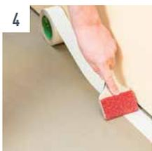
**4** Affix the supplied Sigan tape along walls and protrusions. This provides increased adhesive strength in the edge areas.
