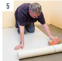
**5** Install the Sigan sheets on butt in the direction of the floor covering to be installed or cut back the overlap of the sheets on butt.
