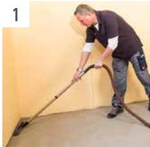
**1** The smoothed substrate, according to DIN 18365, must be sound, level, permanently dry, free of cracks, clean and free of materials that could impair adhesion.
