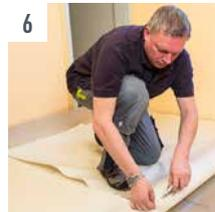
**6** Fit the acclimatized floor covering. Fold back half of the floor covering. Pull the protective paper away from the Sigan 1 horizontally and straight up to the folded back floor covering.
