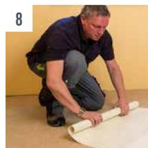
**8** The floor covering can be walked on and used right after bonding. The floor covering can be removed without residues even years later.
