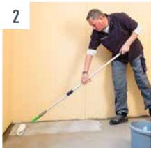
**2** Shake the Planus container well and refill into a clean bucket without diluting it. Apply the ready to use special primer with a fine-pored UZIN foam roller undiluted, uniformly and thin. Allow two dry well ventilated for min. 2 hours.
