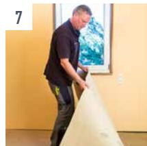
**7** Slide the floor covering without open time onto the Sigan film carrier flat on the floor and roll-out. Proceed accordingly with the 2nd half of the floor covering.
