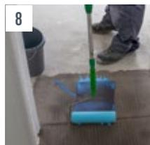
**8** The crack is closed after 1 hour drying. Subsequent work can be continued by applying UZIN PE 360 PLUS primer and allowing to dry for approx. 30 minutes.
