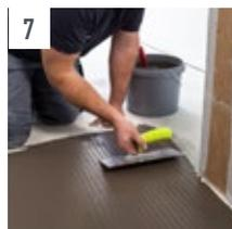
**7** Use a WOLFF smoothing trowel to run over the crack bridge and then apply an even coat of UZIN NC 182.
