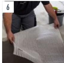
**6** Install UZIN RR 203 with the printed side facing up. Please note that the installation direction of the UZIN RR 203 tiles runs perpendicular to the joint.
