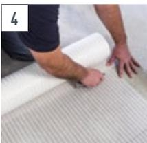
**4** Cut UZIN RR 203 to size and lay aside. NOTICE: joints and cracks have to be covered 30 cm on each side. Alternatively use the pre-cut tile.
