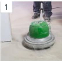
**1** First grind the substrate with a WOLFF grinding machine to remove any materials that could impair adhesion.
